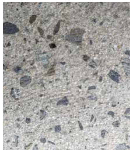
Concrete blasted, scarified, or grinded to an open texture exposed aggregate finish
