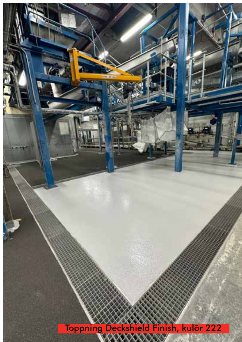
After pumpning Isocrete Industry
