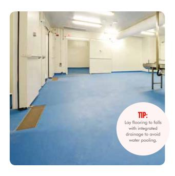
Of the different types of resin flooring systems, one of the most popular hard wearing solutions able to provide the necessary properties is polyurethane. This material combines cement and water-based technologies to produce a mortar that is trowel applied on site to create a very strong and seamless finish. Polyurethane has a high cross-linked density, which makes it a good choice for areas that undergo abusive chemical attack.
