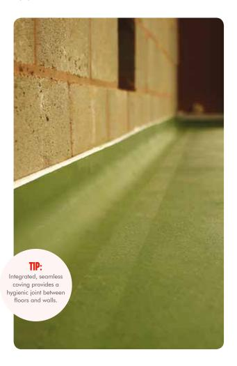
Importantly, polyurethane is much better at resisting thermal shock than other types of resin flooring, as it has a thermal coefficient of expansion similar to concrete. This means that when it is applied over concrete it is able to expand, contract and move with the substrate when the floor is subjected to large temperature changes, like steam cleaning. Floor coatings that do not react with the substrate are much more likely to crack.
